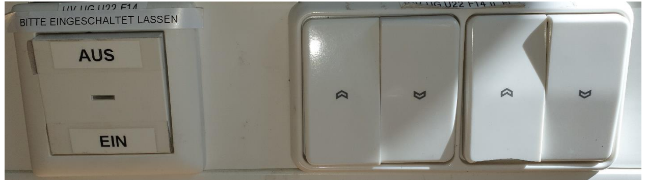
Switch for speakers and screen configuration (up/down) in cable tunnel
